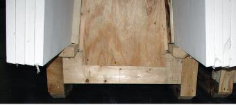
Figure C-2: A-frame shown with runners for box truck movements.
